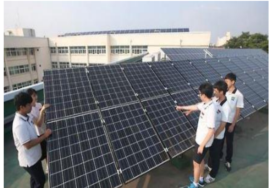
<Solar PV installed on school rooftop>
